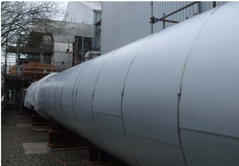
FGR duct from grit arrestor
